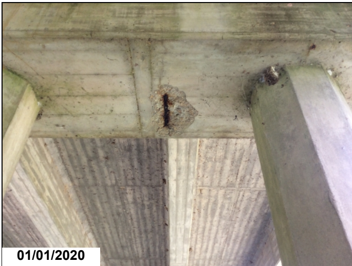
Spall with rebar exposed to bottom of Cap between Piles 3 & 4 @ Bent 14.
