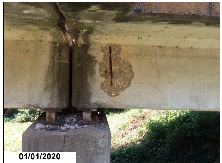
Spall with rebar exposed to Girder 4 @ BOS 16 Right.
