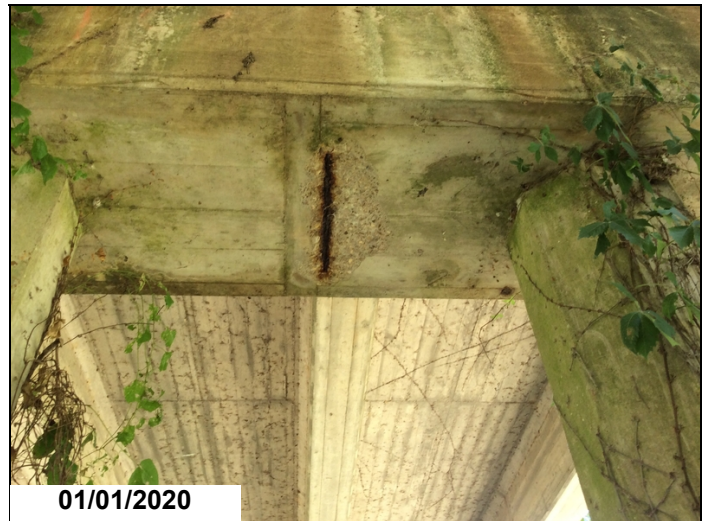
Spall with rebar exposed to bottom of Cap between Piles 3 & 4 @ Bent 12.
