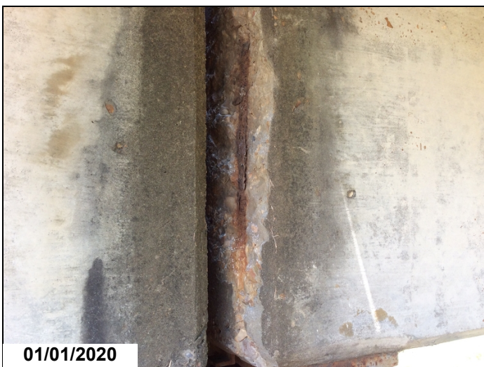
Girder 4 at beginning of Span 9 spalled with 12" of exposed rebar.
