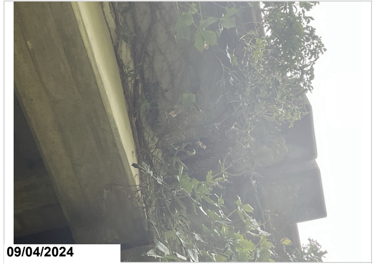
Span 12 left overhang. 1ft rebar 1ft spall
