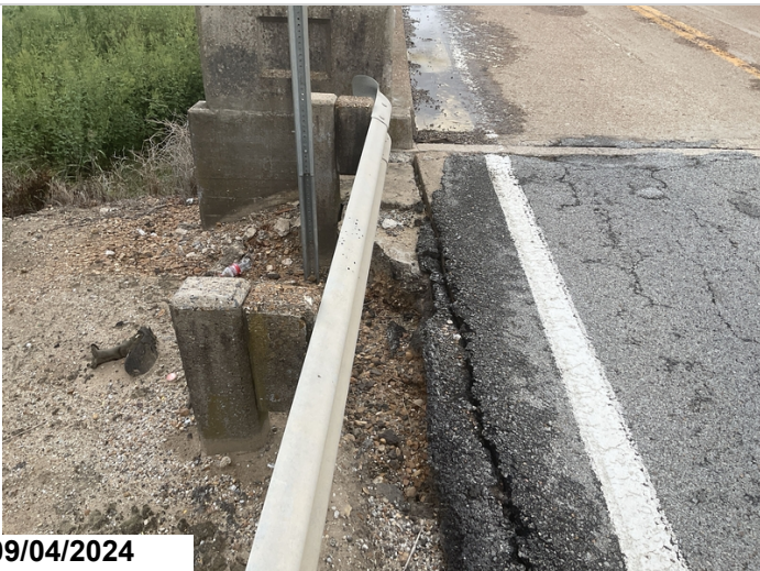
Abutment 1, left. Settlement and erosion at curb
