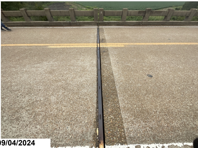
Bent 3. No joint armor ahead side
