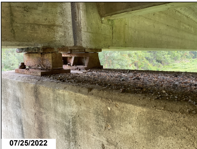
Bent 6 - Fixed Brg. 1, 3 Fixed brg 1.
