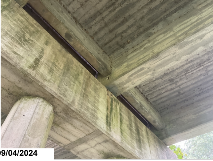
Bent 15, ahead, g2: exp rebar
