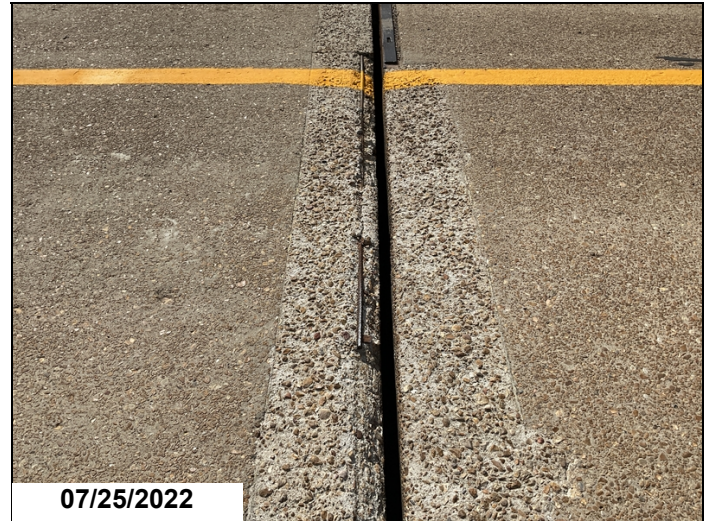
Spalls with rebar exposed to joint @ BOS 11.
