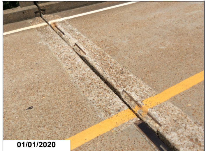
Patched area has spalls with rebar exposed @ BOS 11 Left lane.
