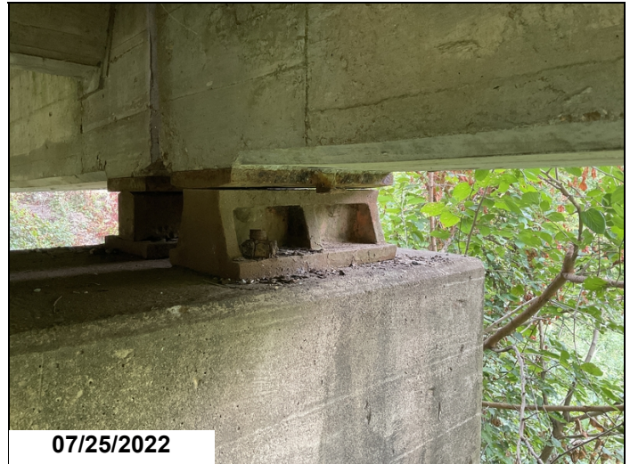
Bearings that are non-bearing: Bent 1 - Fixed Brg.1
