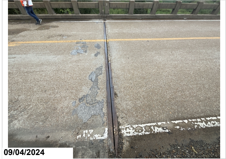
Bent 1. Joint is open, road armor is broken for 15ft
