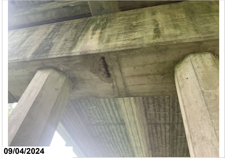
Bent 15 tween piles 3 and 4. 1ft exp rebar
