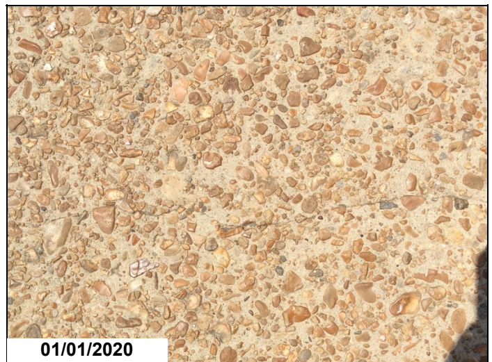
Unsealed transverse cracking to Deck @ Span 5.
