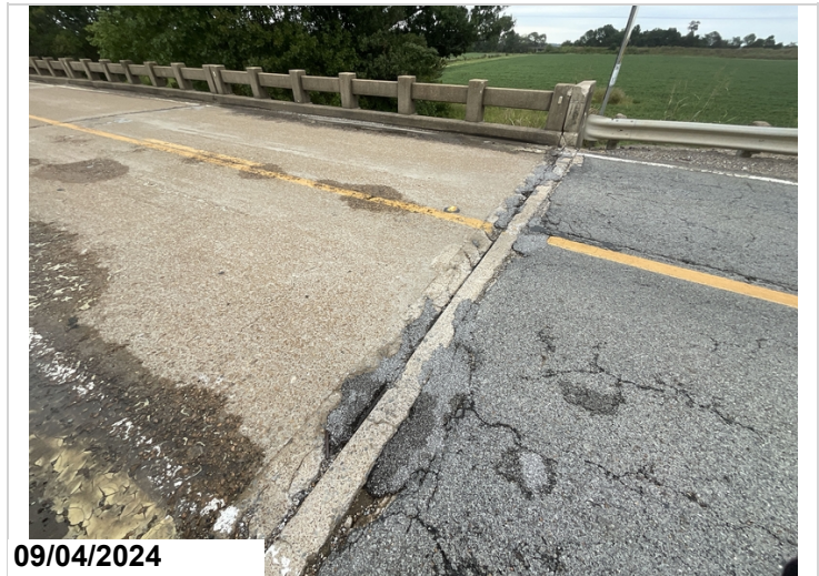
Abutment 1. The deck is spalled adjacent to the headwall with exposed rebar throughout. 9sf rebar. Remaining deck width x1' spalled
