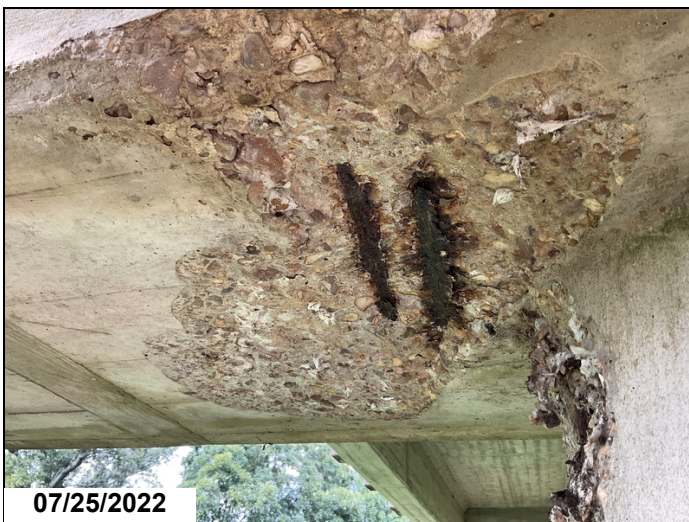
Spalls with rebar exposed to caps at Bents 5, 12 & 14. Bent 5, between piles 4 & 5.
