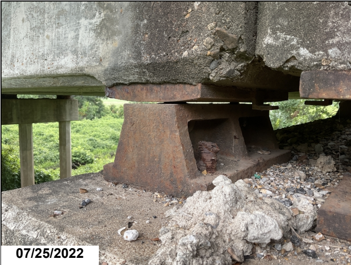
Bent 2 - Fixed Brg. 1 & 4 Moveable Brg. 1 Fixed brg 1
