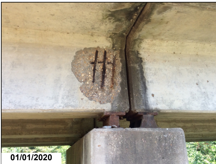
Spalls with rebar exposed to Girder 4 @ EOS 3.
