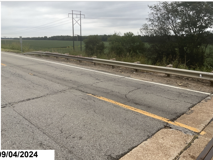
Bridge rail transitions are in good condition with only minor surface corrosion.
