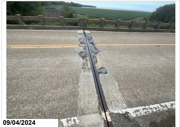
Deck at bent 2 has spalling on both sides of joint with exposed rebar and unsound patches. 2ft cs3 rebar. 2x 15 cs3 spalling/patch. Right gutter has 1x2 spall at bos 3
