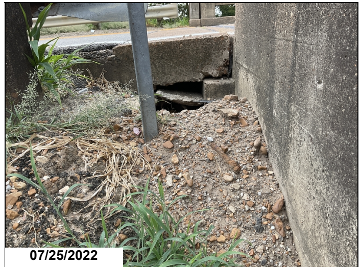
Approach roadway at Abutment 2 has erosion 8" below and 8' back under roadway.
