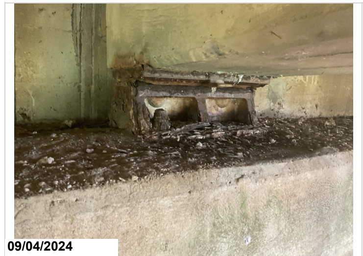
Abutment 1, bearing 2. Heavy corrosion.all have cs3 corrosion. This is worst case
