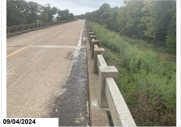
The bridge railing has minor vertical cracks and spalls throughout.
