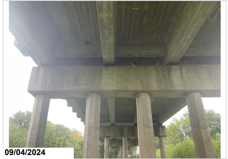
Bent 2, back,g2 crack with rust
