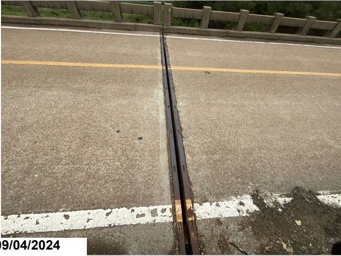
Bent 6, joint armor is cracked and broken in numerous places. Loud when cars pass. Bent 7 similar
