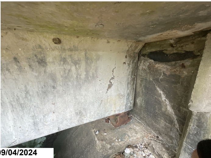
Abutment 1, g1. Spall 1ft
