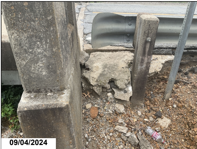
Abutment 1: has rotated ahead with settlement at the approach.
