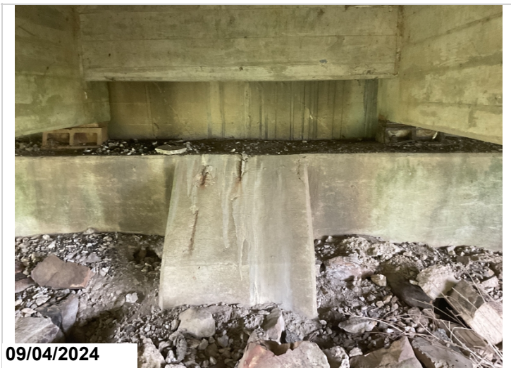
Abutment 1 backwall, center: cracking 4ft exp. Rebar 2'
