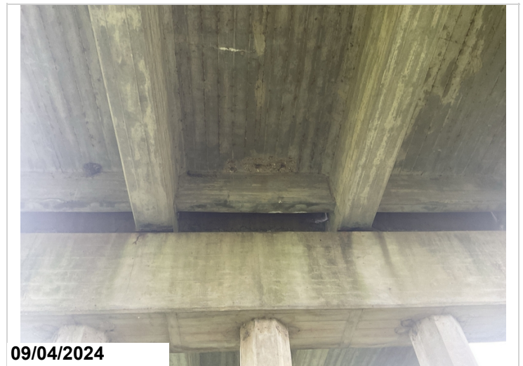
Span 2, bent 2, bay 2: spall
