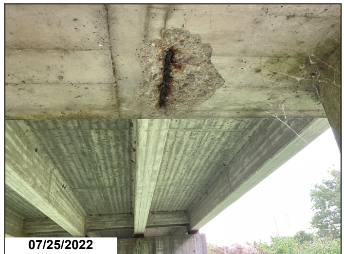
Spalls with rebar exposed to caps at Bents 5, 12 & 14. Bent 14 between piles 3 & 4.
