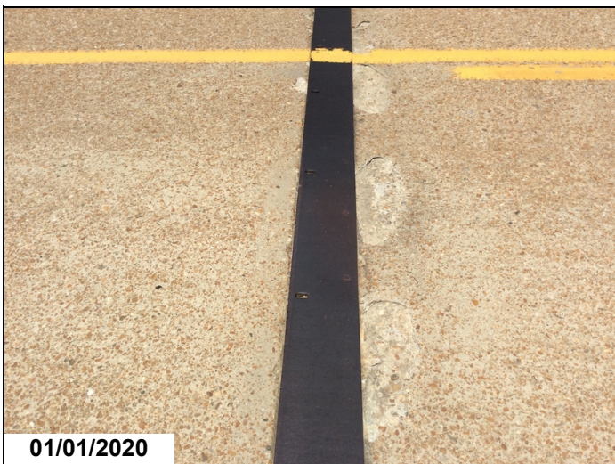
Spalls and delaminated areas along joints @ EOS 4 & BOS 5
