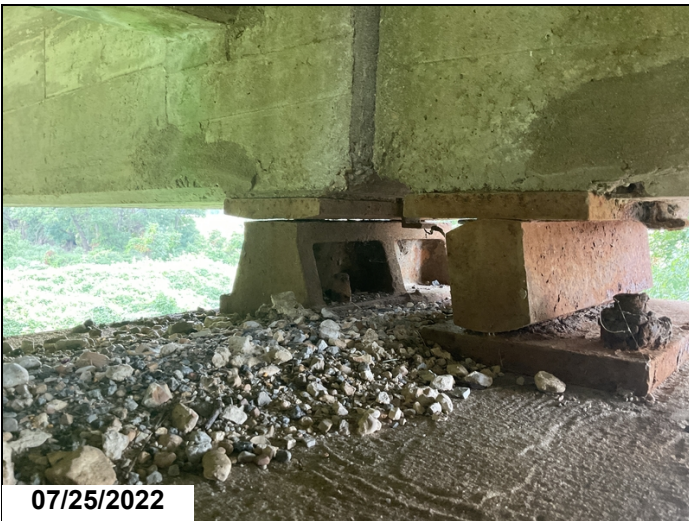
Bent 2 - Fixed Brg. 1 & 4 Moveable Brg. 1 Fixed brg 4.
