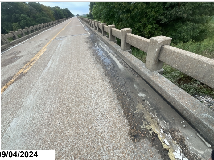
Typical abrasion in gutters
