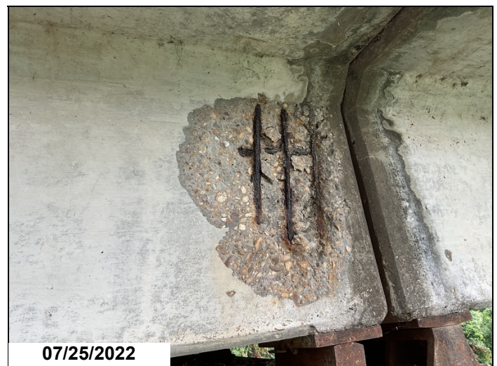
Spalls with rebar exposed to girders at Spans 3, 5, 6, 9, 15 & 16. Girder 4, end of span 3.
