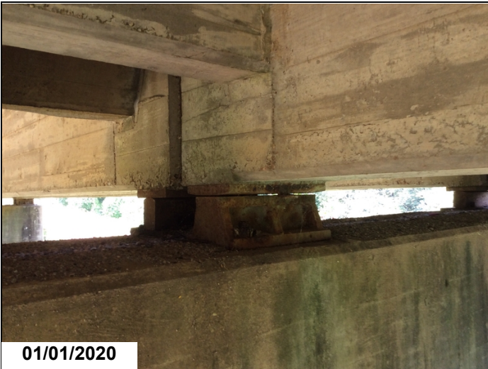
Fixed Bearing 2 @ BOS 4 is non bearing.
