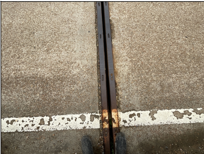
Bent 5 is cracked and sounding when cars pass
