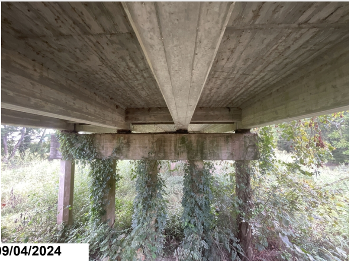
Bent 15 bearings. All cs3
