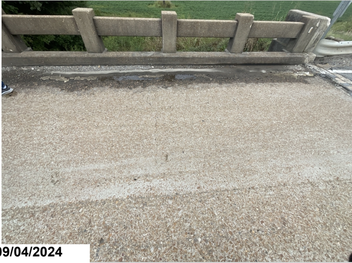
Typical transverse cracks
