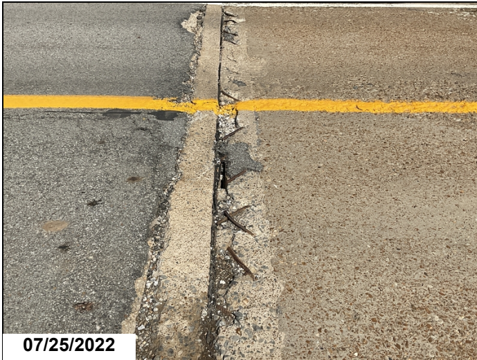
Spalls and delaminated areas along all joints. Abutment 1.
