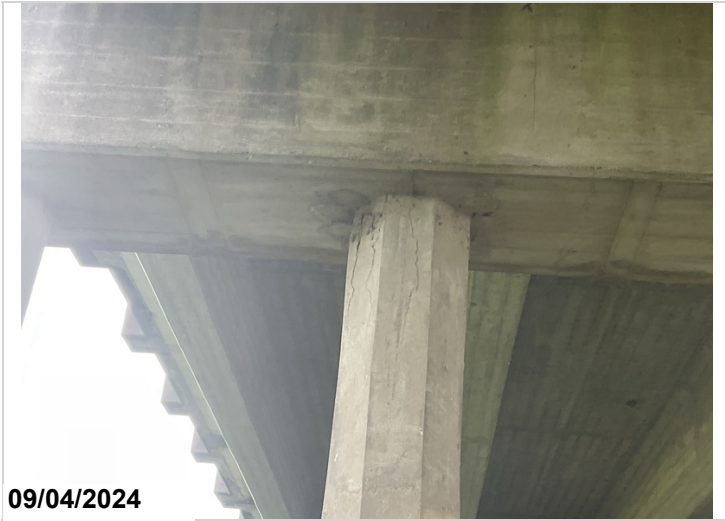
Bent 2, pile 2: heavy vertical cracks
