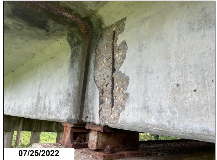
Spalls with rebar exposed to girders at Spans 3, 4, 5, 6, 9, 15 & 16.
