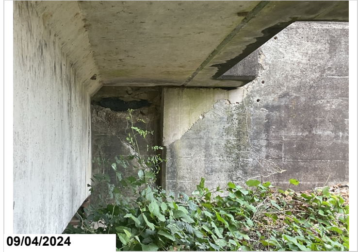
Abutment 1 left. 2ft spall and large crack
