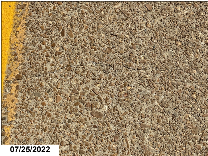
Unsealed transverse cracks to deck @ all spans.
